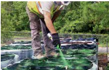
IMAGE B: Uniaxial geogrid rolls should be color-coded prior to removing roll labels.
