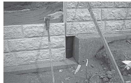
IMAGE G: Upper leveling pad offset 9 in.
