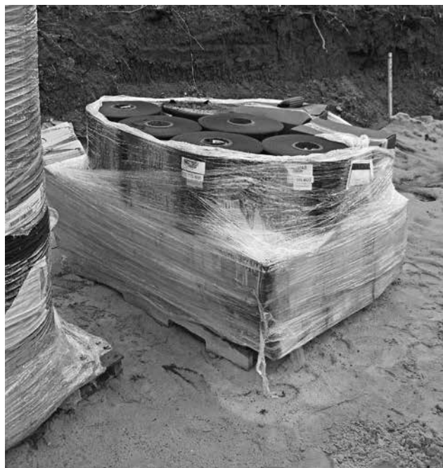
Palletized component materials upon arrival at site.
