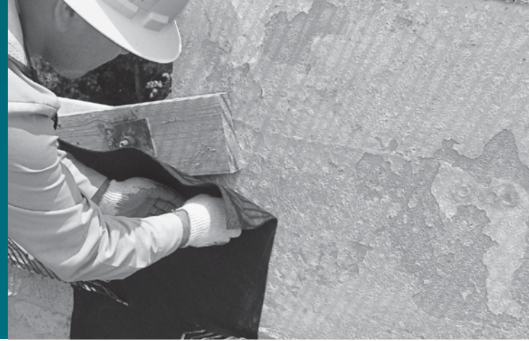
IMAGE L: Placement of filter fabric at ARES® vertical joint.
