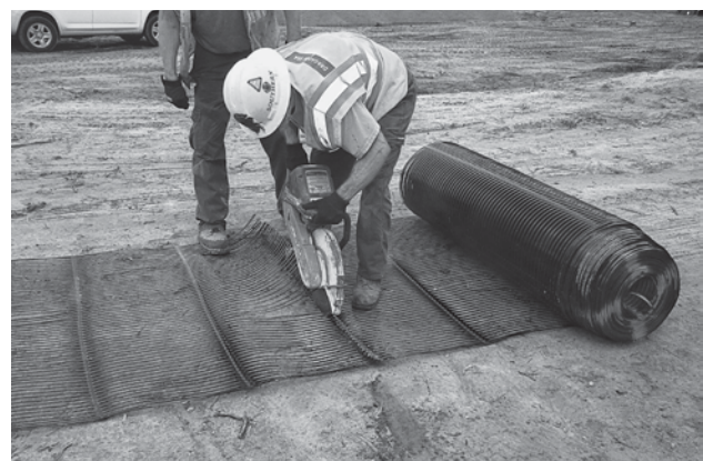
IMAGE D: Safe cutting of geogrid may be accomplished with a variety of cutting tools. Care should be taken to avoid cutting the transverse bar.
