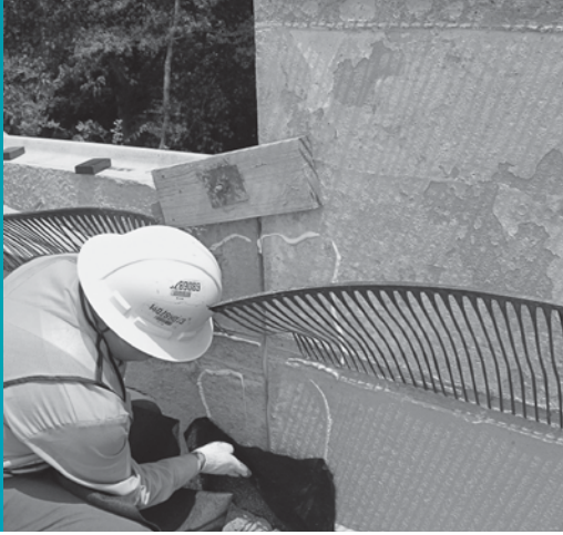
IMAGE K: Preslit fabric at geogrid elevations.
