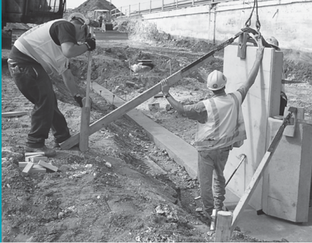
IMAGE H: Bracing of ARES® panels.
