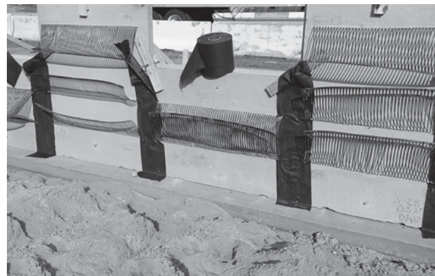
IMAGE N: Filter fabric at vertical joint of ARES panels.
